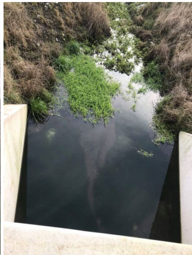
SWML 4 Outfall Headwall
