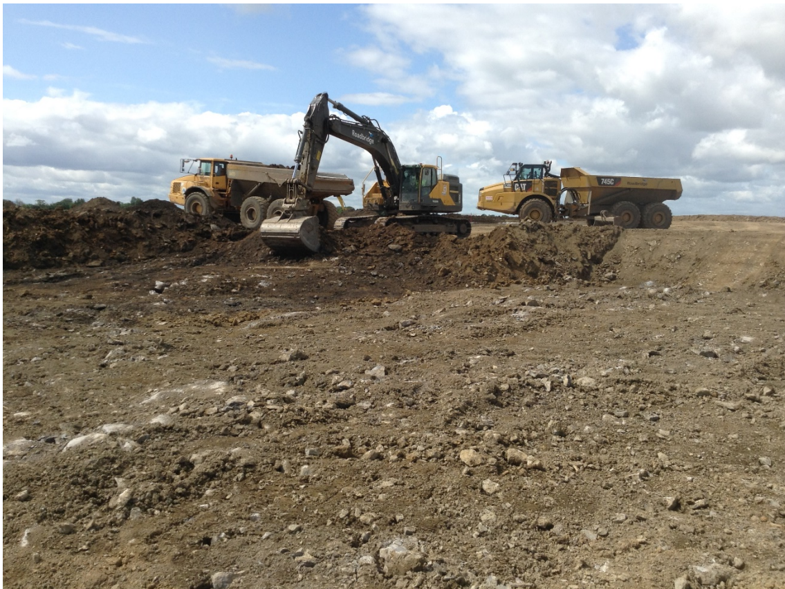
Sectional stockpiling and surfacing along APEC 5 area
