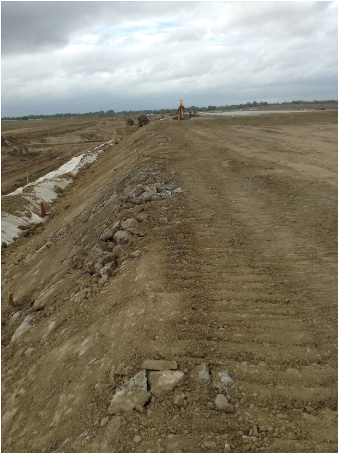
View West at Material Stockpile
