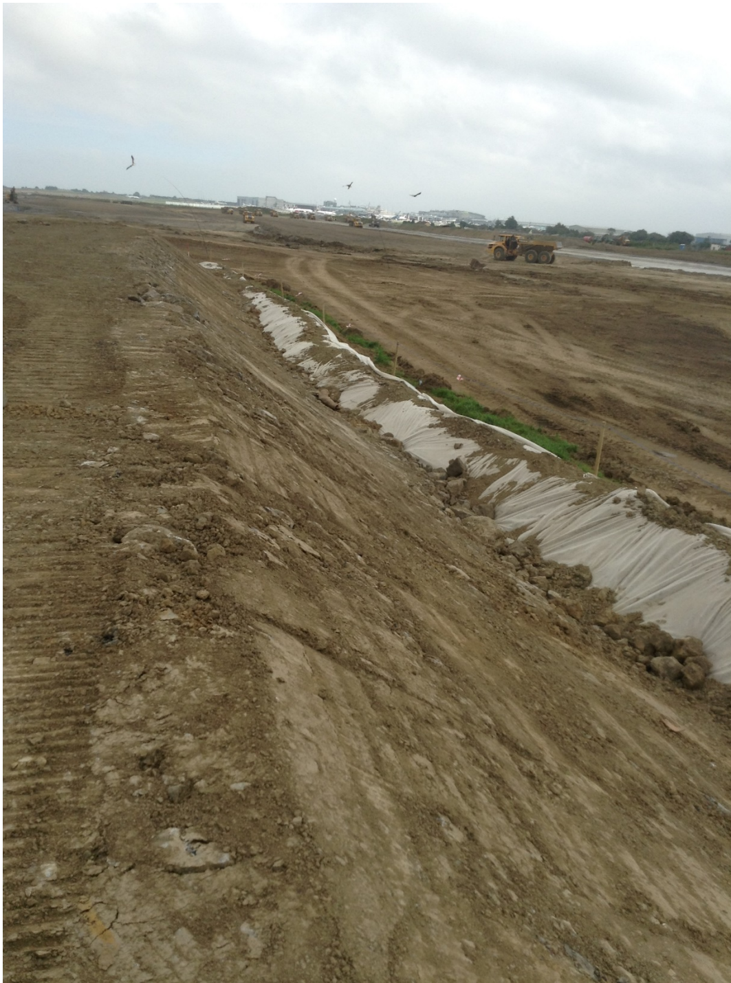
View South East at Material Stockpile
