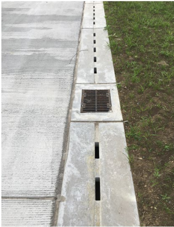
Figure 4-3: Paved Area Slot Drain at Edge of Runway and Taxiway
